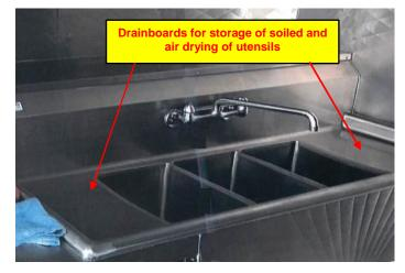
Fixed 3-compartment set up with drainboards
