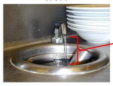
Air gap between water supply line and flood rim of receptacle
