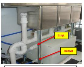
Water tank under 3-comparmtent sink in unit
