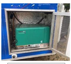
Generator installed in exterior compartment of unit
